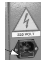
SHOCK HAZARD POWER SOCKET
